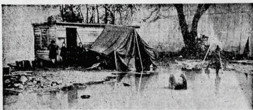
NO TENTING LAST NIGHT at this Ferry Street bridge home. Waters lapped at the entrance and rose steadily two feet more after this photo was made. A family is leaving wooden structure behind tent.
