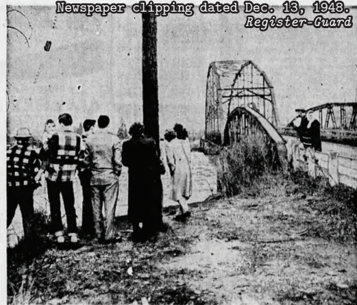
OVERLY ANXIOUS SPECTATORS flocked to vantage points to watch the turbulent Willamette River on her annual rampage. Many had understandable interest in their dwellings but thousands on "sight-seeing tours" merely hampered work of authorities. This group watches swirling waters below Ferry Street Bridge.
