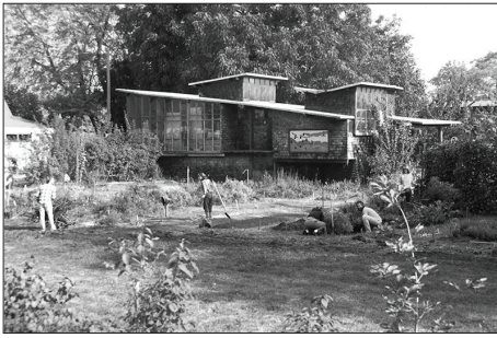
Circa late 1970s, the newly established Urban Farm takes shape around the Graduate Shelter. Note the completed Fine Art Studio building C in the background. UO College of Design
